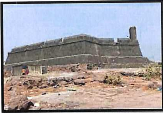
Figure 2.24 Worli fort built by Britishers
