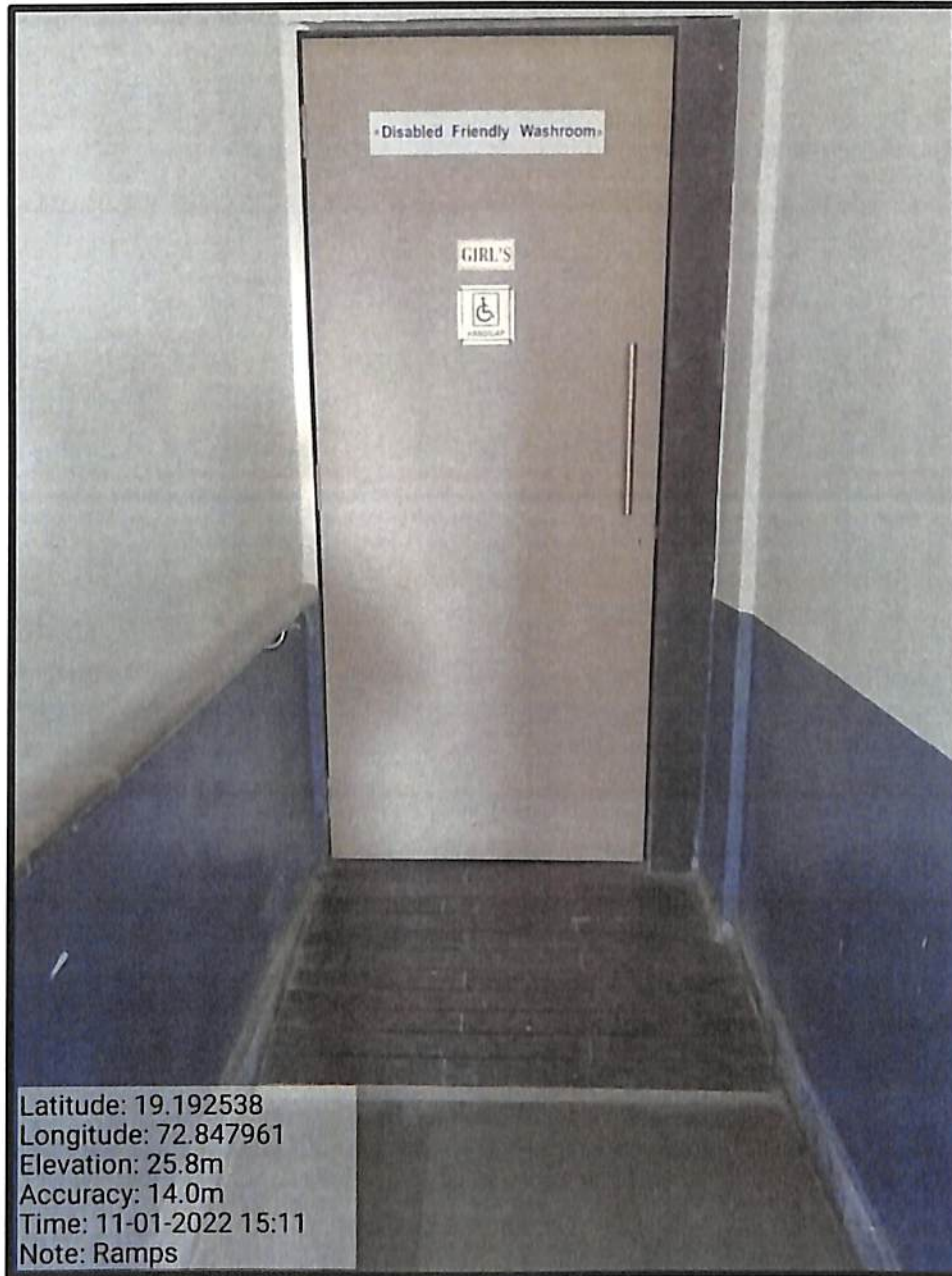
Ramps with adequate slope at entrance of washroom
