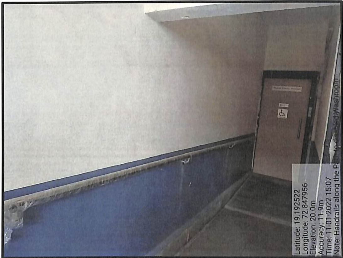
Handrails installed at entrance path of washroom
